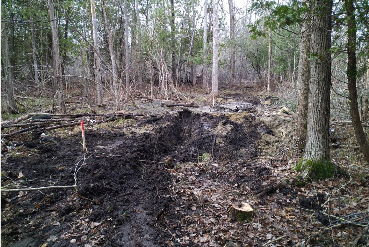
Photo 21: Location of Test Pit No. TP-20 to TP-22, Facing North from TP-22
