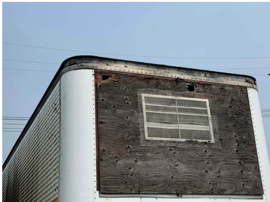
Photo 12: Structure within the study area, holes indicate it has potential to be used as a roost for bats and barn Swallows, June 29, 2023.
