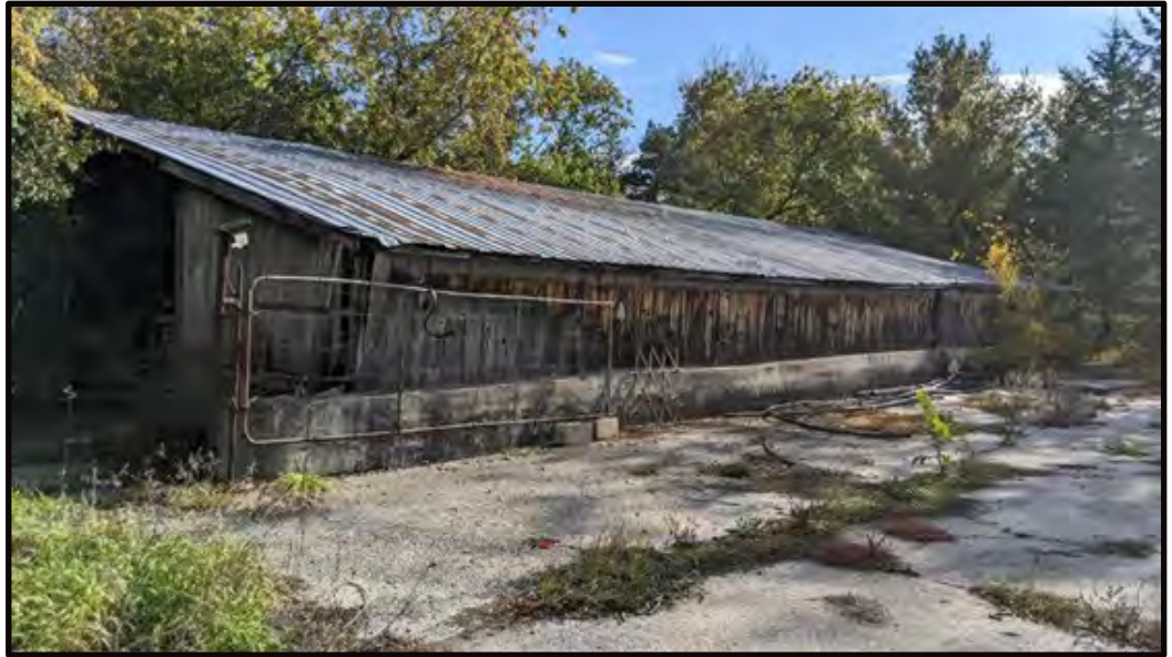
Photo 19: Decommissioned structures are present within the property. Structures such as this have potential to house birds species such as Barn Swallow.
