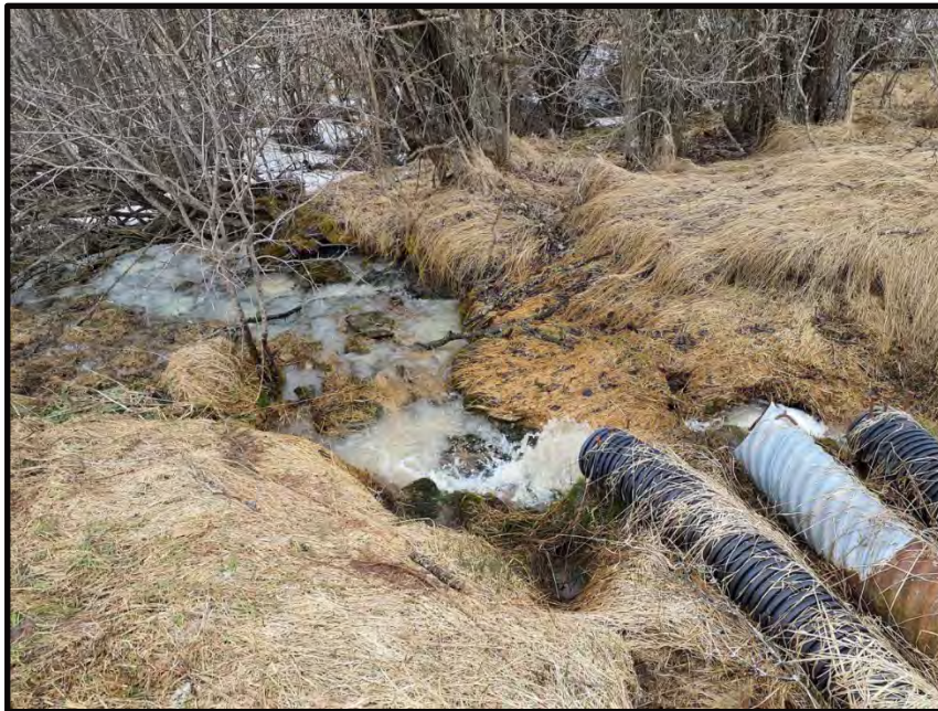
Photo 13: Tile drains diverge water from the Annual Row Crop (OAGM1) Community into Wetland-2. Observed on April 11th, 2023.
