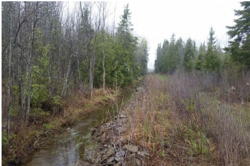
Photo 23, 8-May-17 – MMD2, Looking SW
