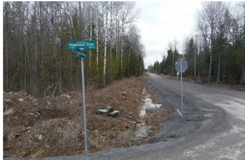
Photo 7, 12-Apr-17 – Ridgemont Dr. Drainage Ditch, Looking NW
