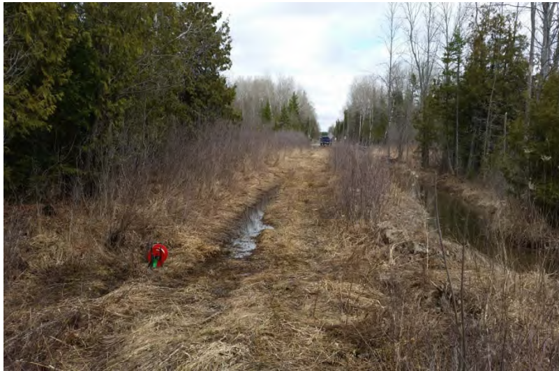
Photo 5, 12-Apr-17 – Location of Abandoned Channel at MMD2, Looking NE
