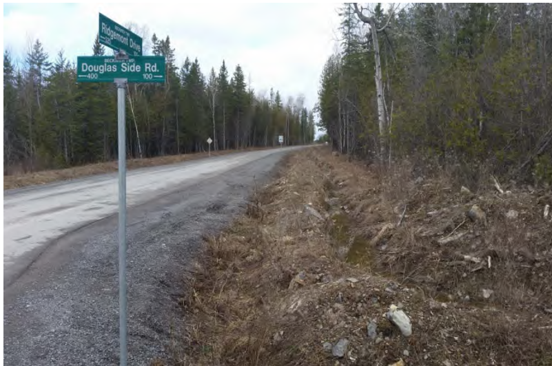
Photo 7, 12-Apr-17 – Ridgemont Dr. Drainage Ditch, Looking NW
