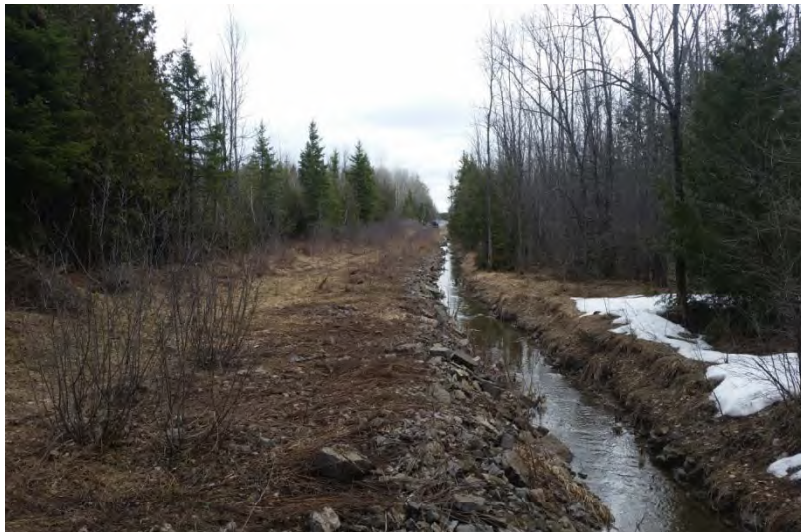
Photo 11, 12-Apr-17 – MMD2, Looking NE
