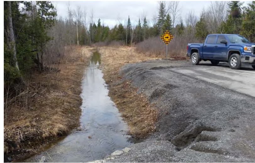
Photo 10, 12-Apr-17 – MMD2 At Edge of Douglas Side Road, Looking SW
