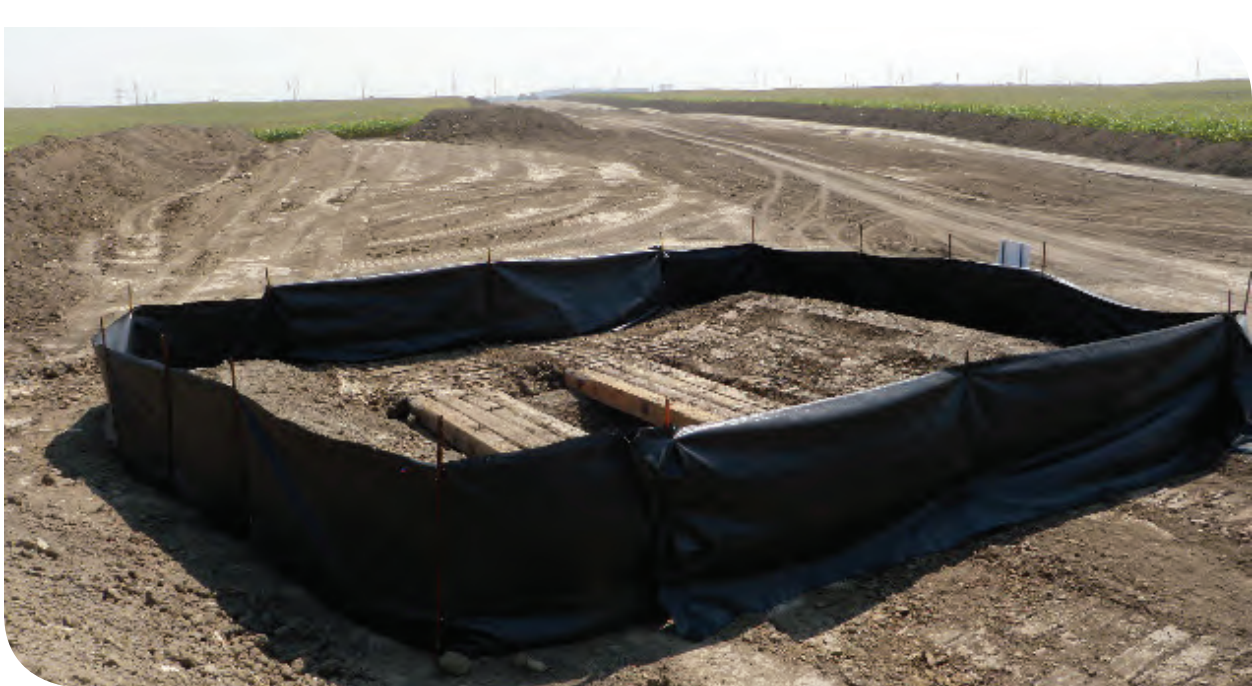
Cleaning station at construction site.
