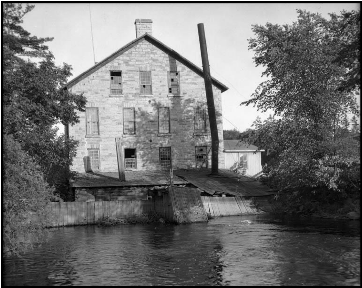
Figure 18: Former Blakeney Woolen Mill, on the pond above the bridge near town. Source: Library and Archives Canada, Colborne Powell Meredith, aO26959.
