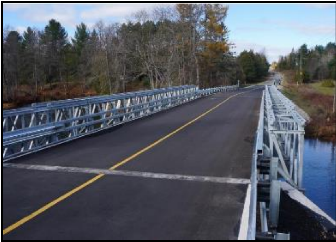
Figure 6: Lanark Highlands modular bridge. This bridge is the same design as the replacement bridge proposed for the Blakeney crossing. Source: [Acrow], n.d.
