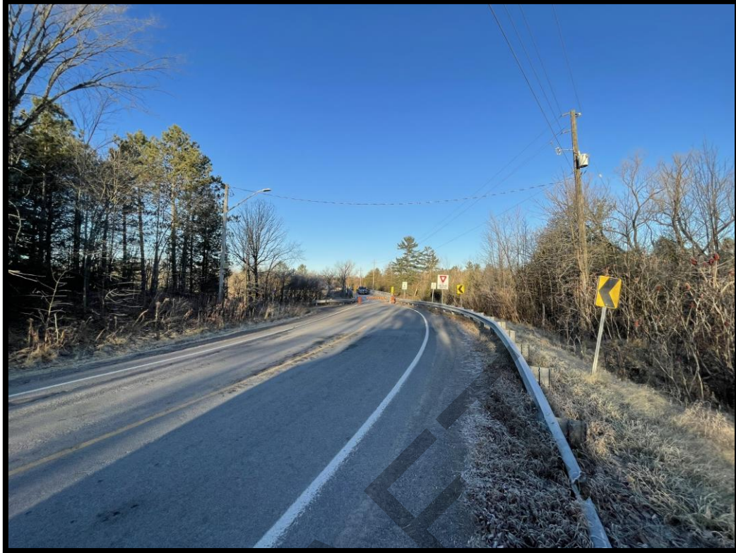
Figure 3: Eastern side approach to the bridge. (MH1149-D003)
