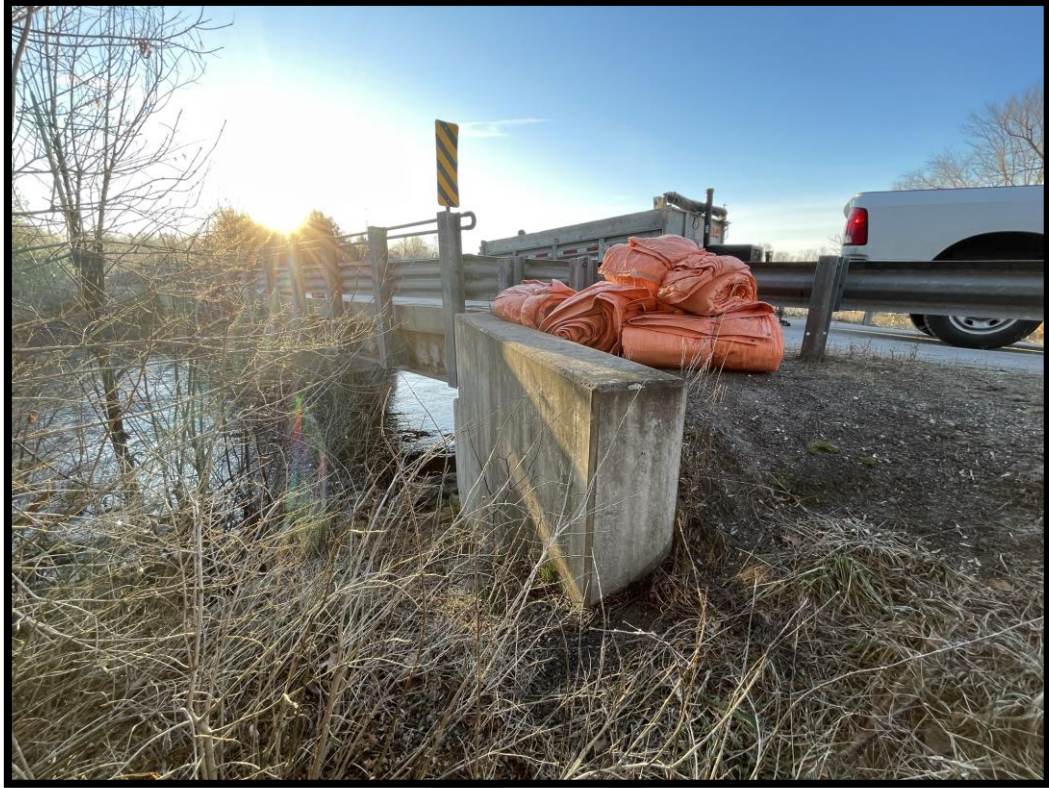
Figure 7: Bridge support on western side. (MH1149-D011)
