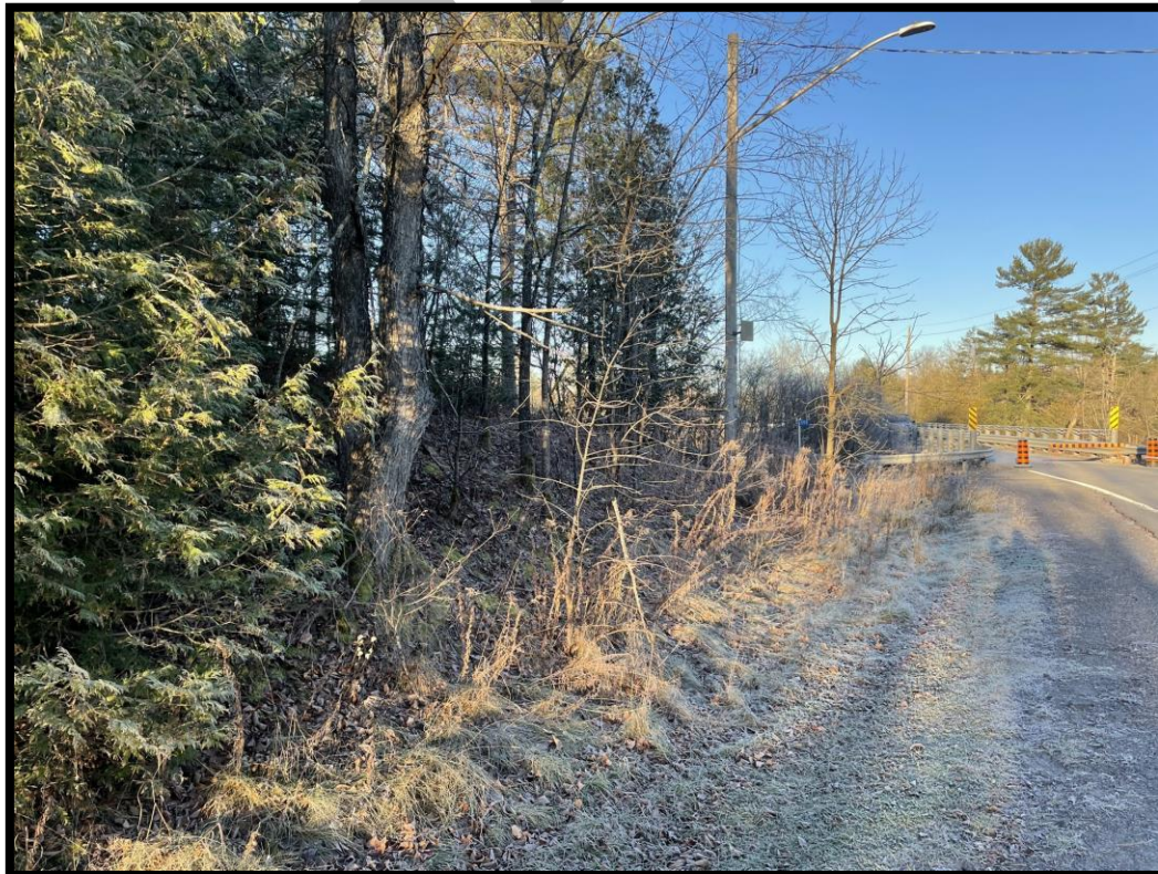
Figure 14: Artificial berm on southern side of the road, approach to the eastern side of the bridge. (MH1149-D004)
