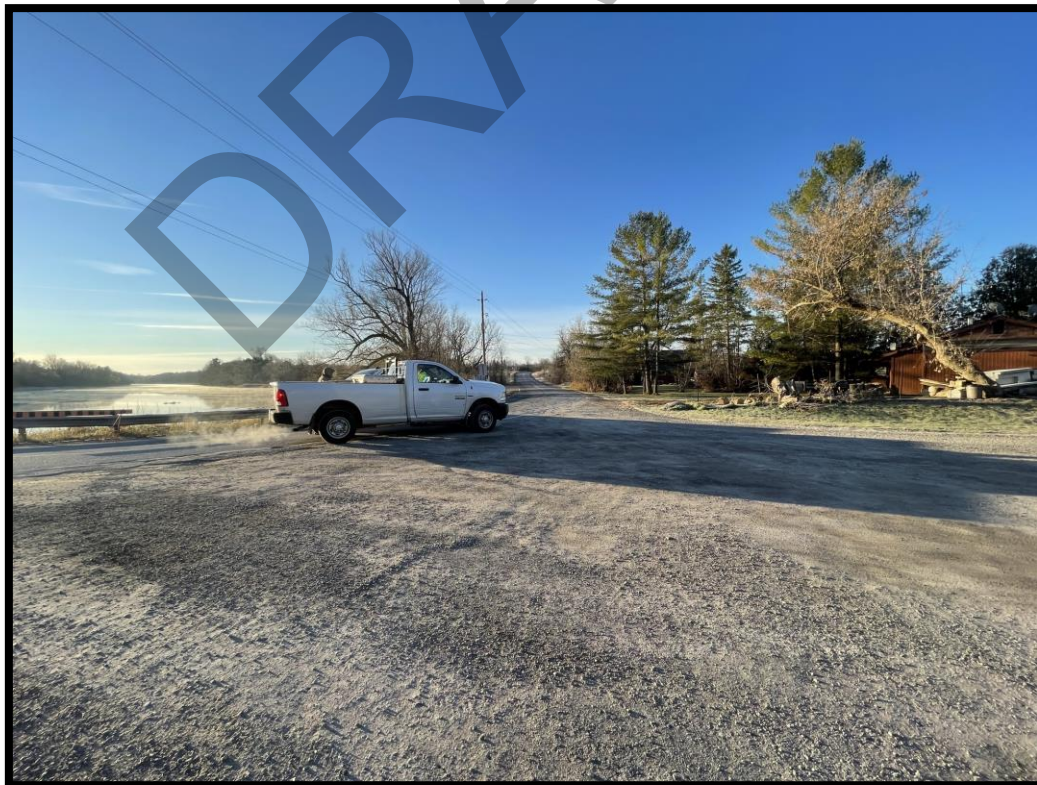
Figure 16: Gravel driveway into park on the western side of the bridge. (MH1149-D013)
