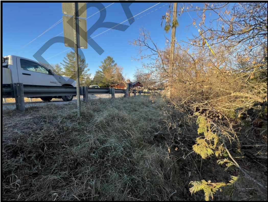
Figure 8: Embankment for road construction on edge of bridge. (MH1149-D012)
