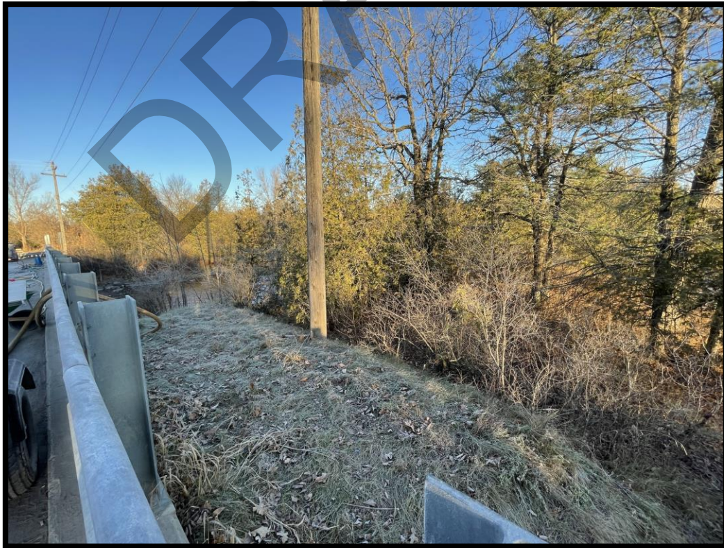
Figure 6: Embankments and bridge support abutments on bedrock. (MH1149-D009)
