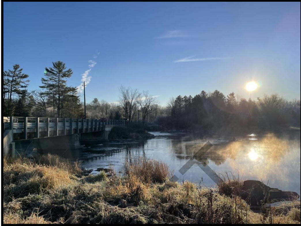
Figure 11: General view of the study area, bridge crossing the Mississippi River, with marshy area along river in foreground. (MH1149-D017)
