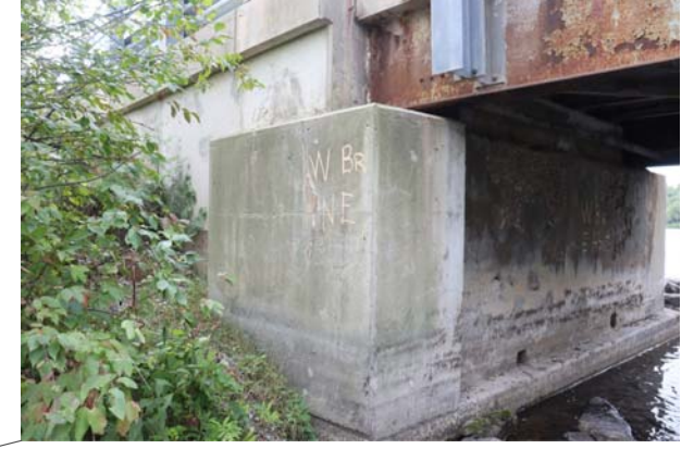
NORTH RETAINING WALL EAST ABUTMENT WEST BRIDGE BETWEEN WEST & MIDDLE BRIDGE
