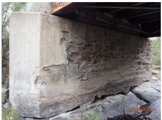
WEST ABUTMENT WALL EAST BRIDGE
