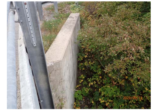
SOUTHEAST WING/RETAINING WALL
