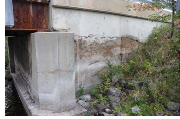
SOUTH RETAINING WALL BETWEEN WEST & MIDDLE BRIDGE
