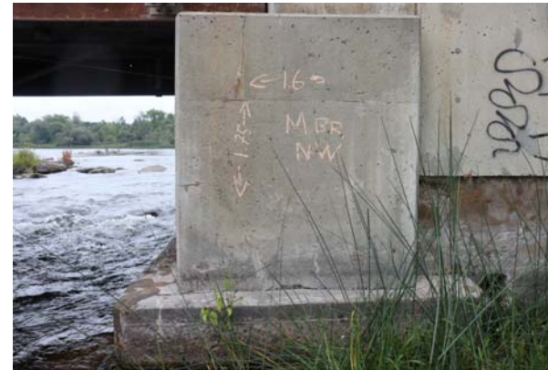
NORTHWEST ABUTMENT/WING WALL MIDDLE BRIDGE
