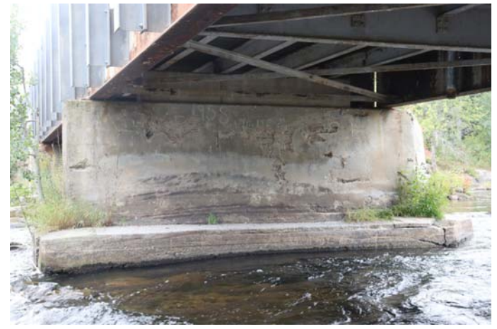
WEST SIDE PIER (MIDDLE BRIDGE)
