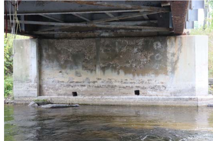
EAST ABUTMENT WALL (WEST BRIDGE)
