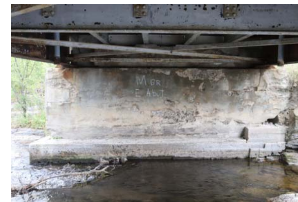
EAST ABUTMENT WALL MIDDLE BRIDGE
