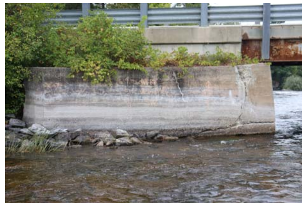
SOUTHWEST RETAINING WALL MIDDLE BRIDGE SOUTH ELEVATION
