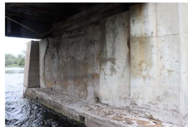
WEST ABUTMENT WALL MIDDLE BRIDGE
