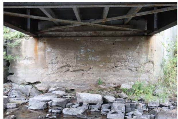
EAST ABUTMENT WALL EAST BRIDGE
