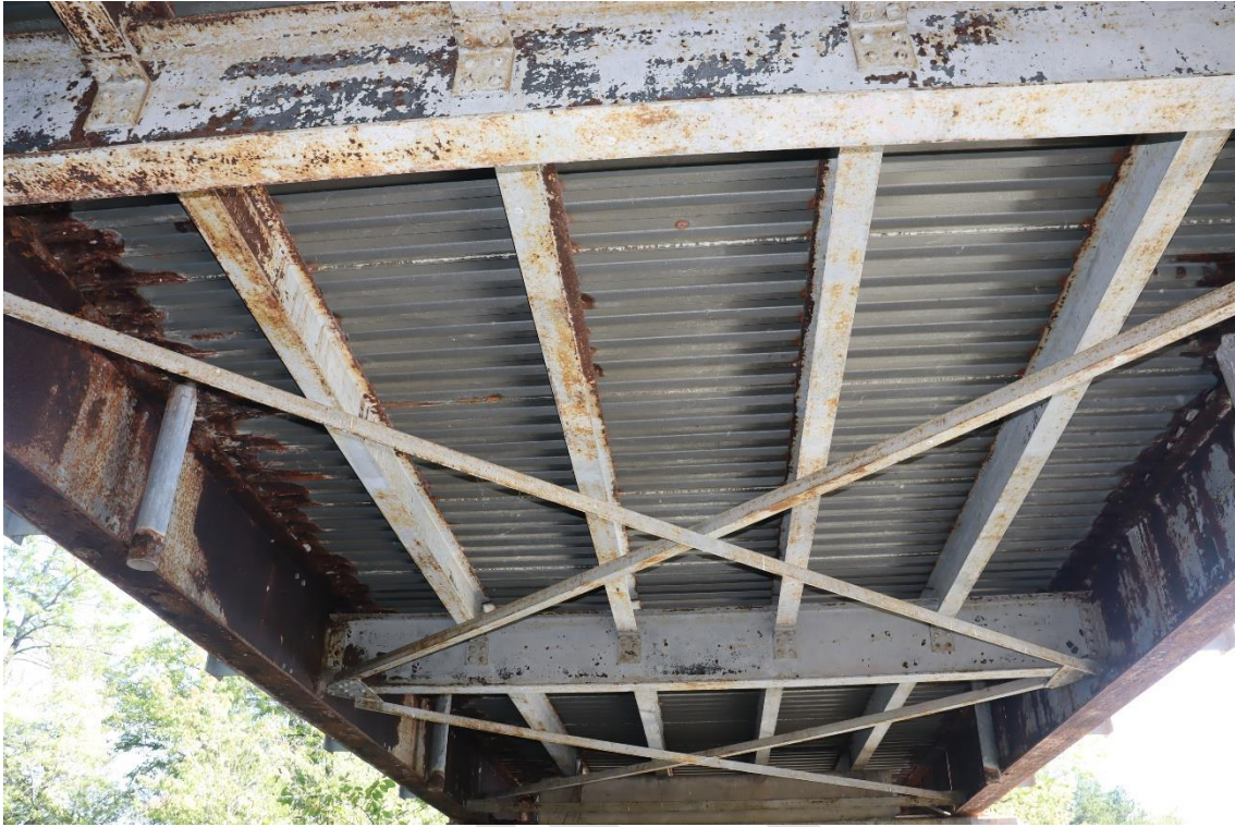
Image 49. Soffit of west span of west bridge facing east
