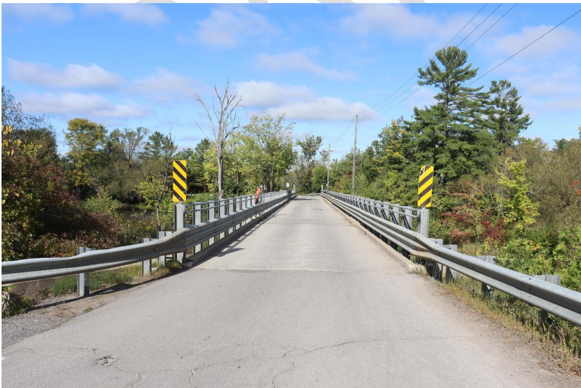
Image 2. East approach of east bridge
