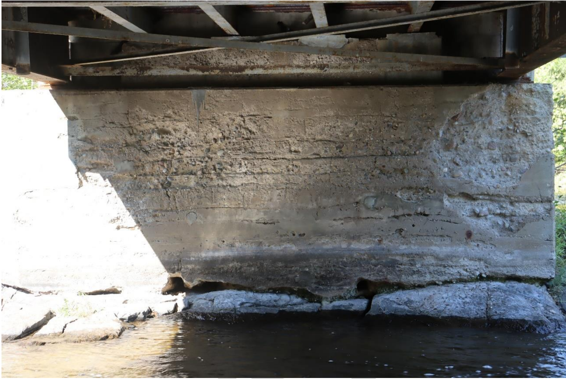
Image 13. West abutment of east bridge
