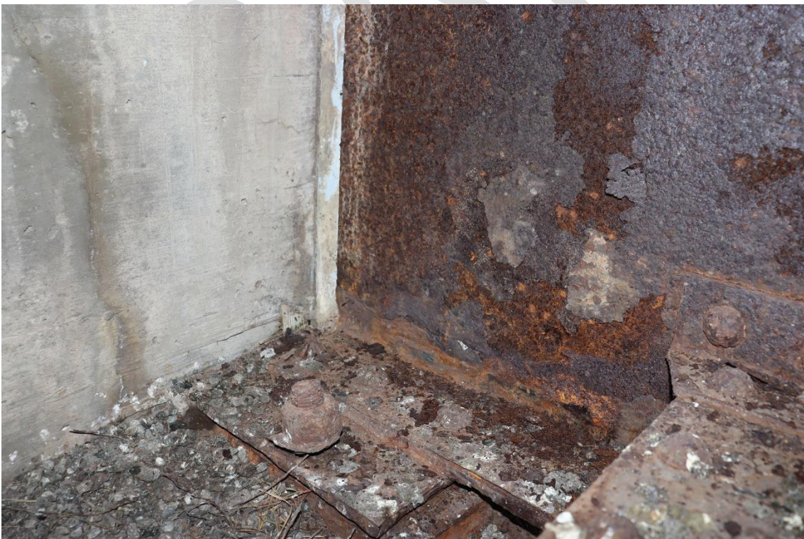
Image 16. Typ. abutment bearing of girders of east bridge
