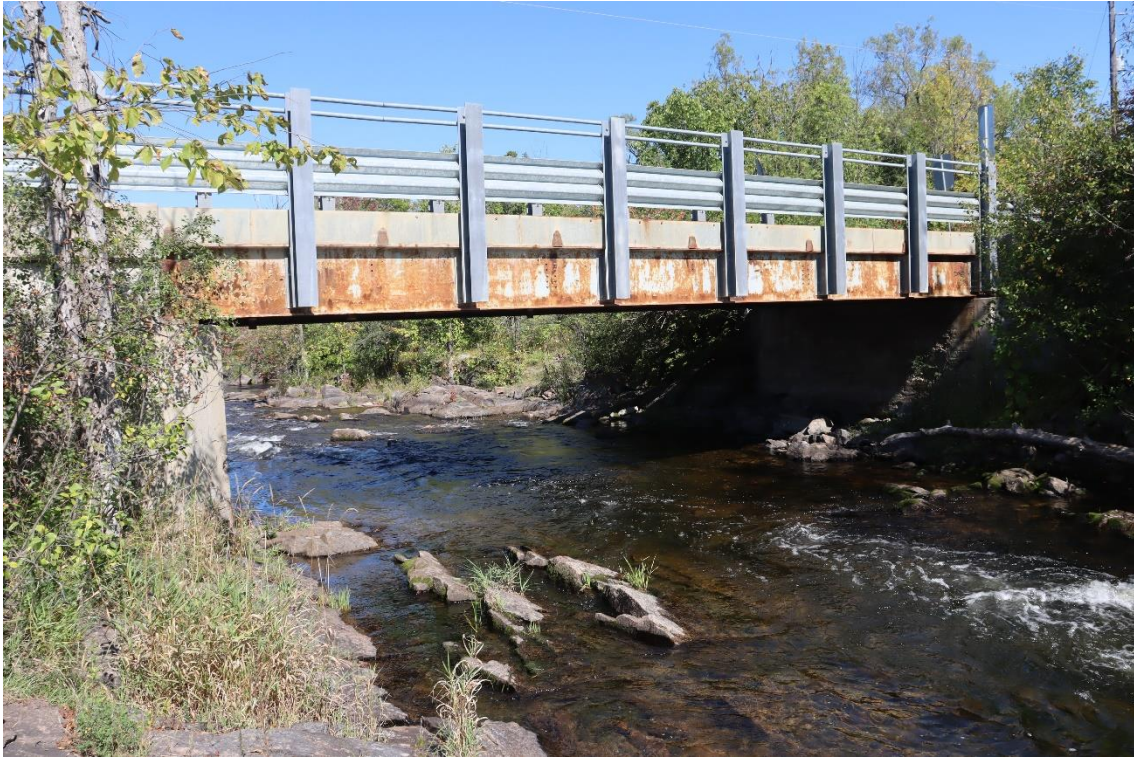
Image 1. South elevation of east bridge
