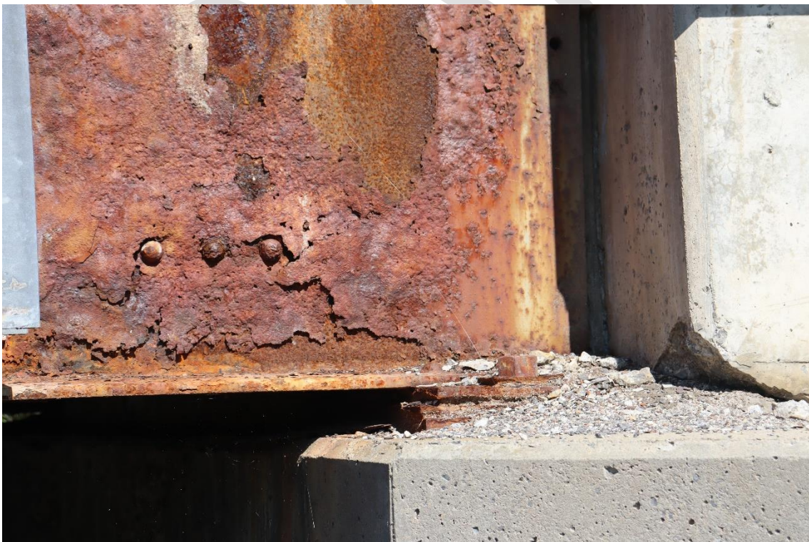
Image 23. Exterior face south girder on east abutment of west bridge
