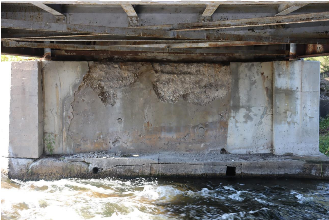
Image 28. West abutment of middle bridge
