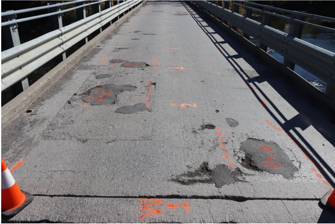
Image 28. West end of west bridge deck condition survey
