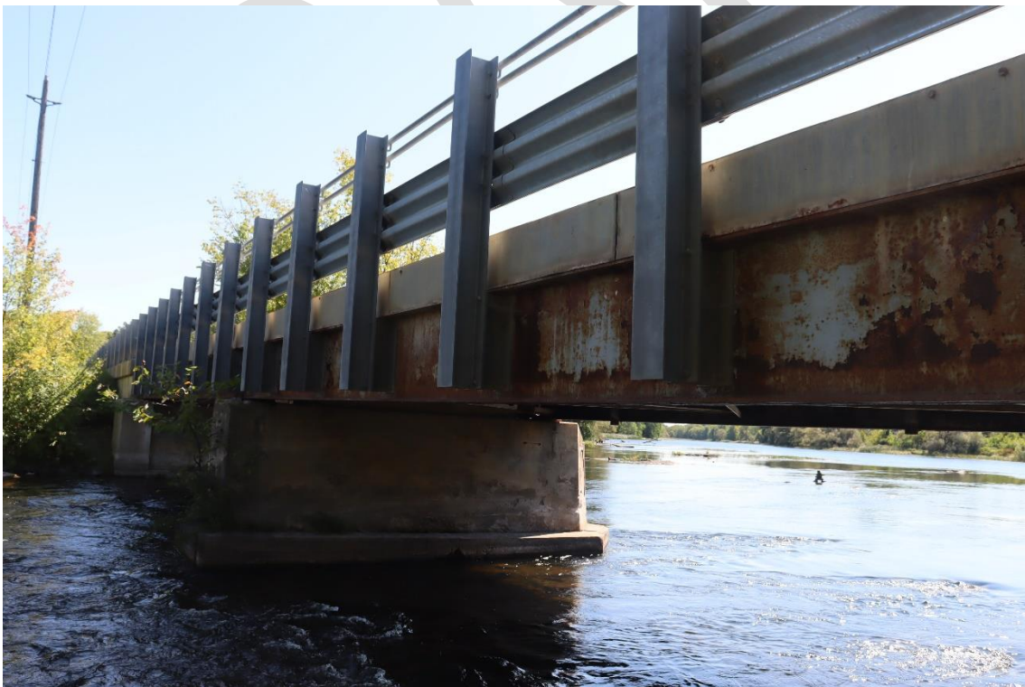
Image 18. North elevation of west bridge
