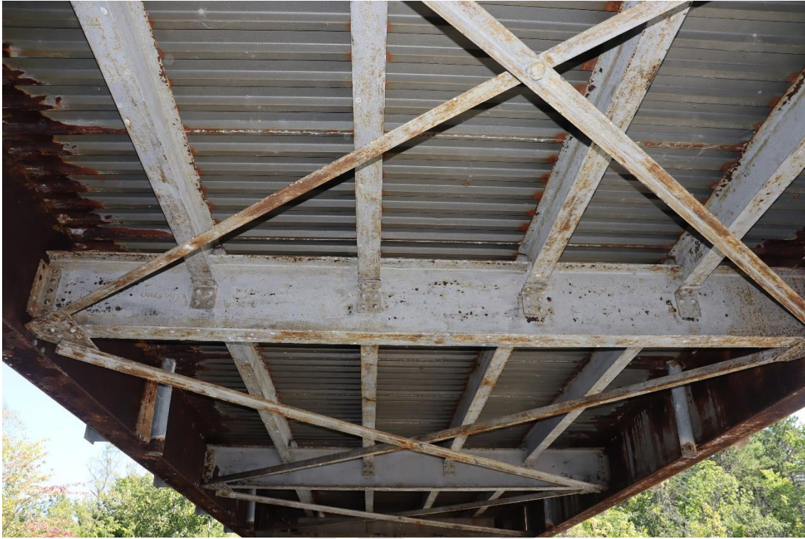
Image 12. Soffit & floor system of west span of middle bridge facing east
