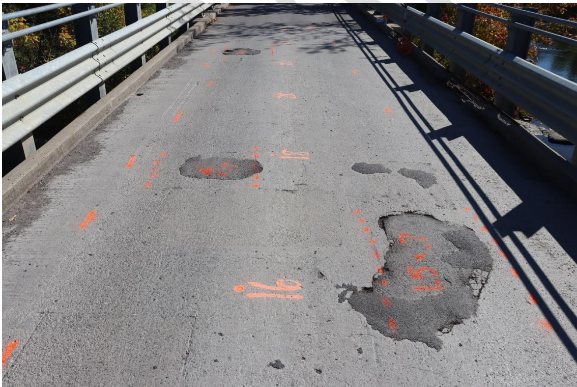
Image 29. East end of west bridge deck condition survey
