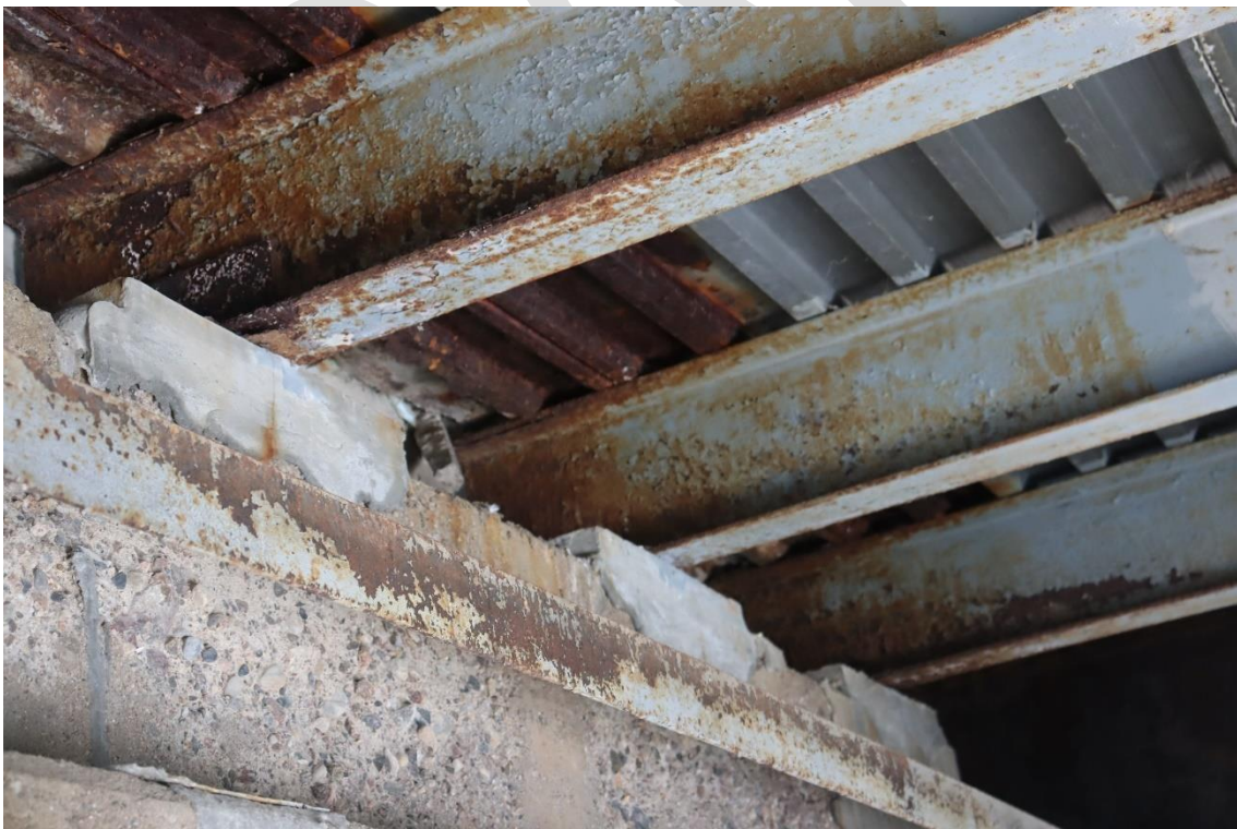
Image 3. Typ. condition of stringer east end of east bridge
