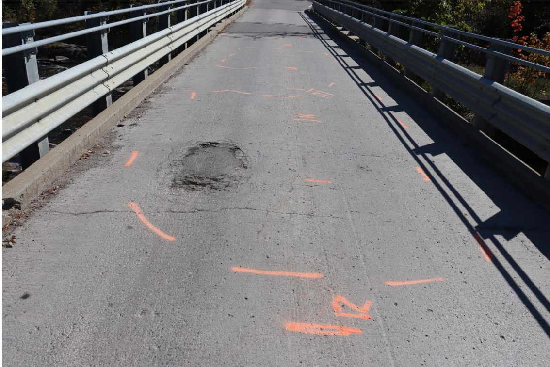
Image 30. Middle to east end of middle bridge deck condition survey
