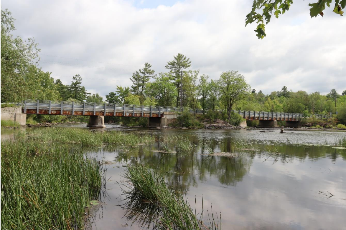
Image 1 Upstream view of Blakeney Bridge
