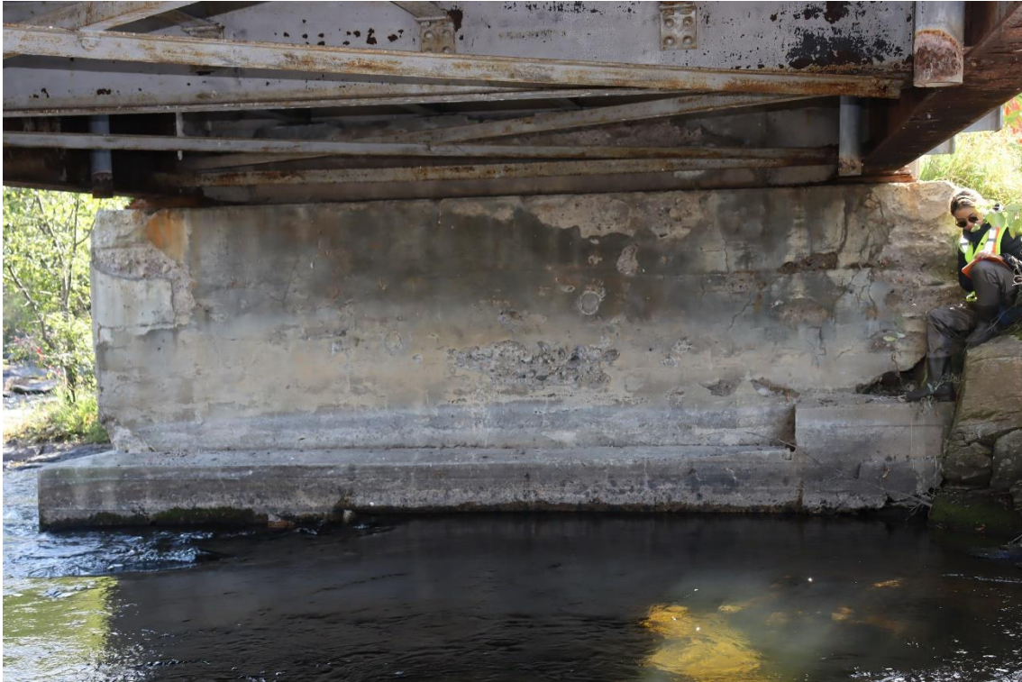
Image 8. East abutment of middle bridge
