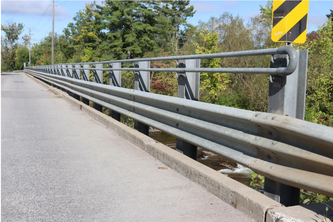
Image 3. Typ. railing system on east bridge
