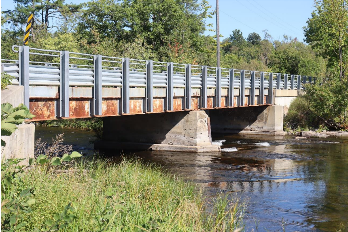
Image 17. South elevation of west bridge
