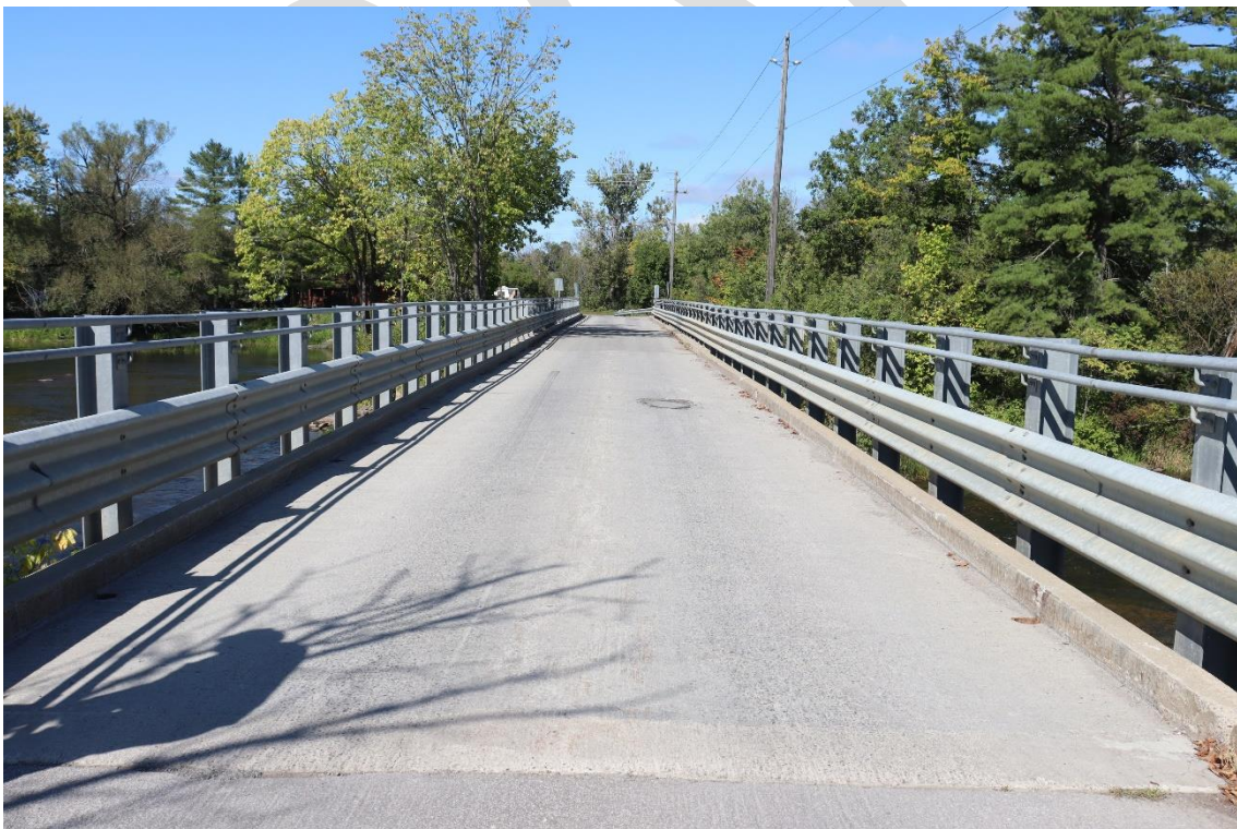
Image 18. East approach of middle bridge
