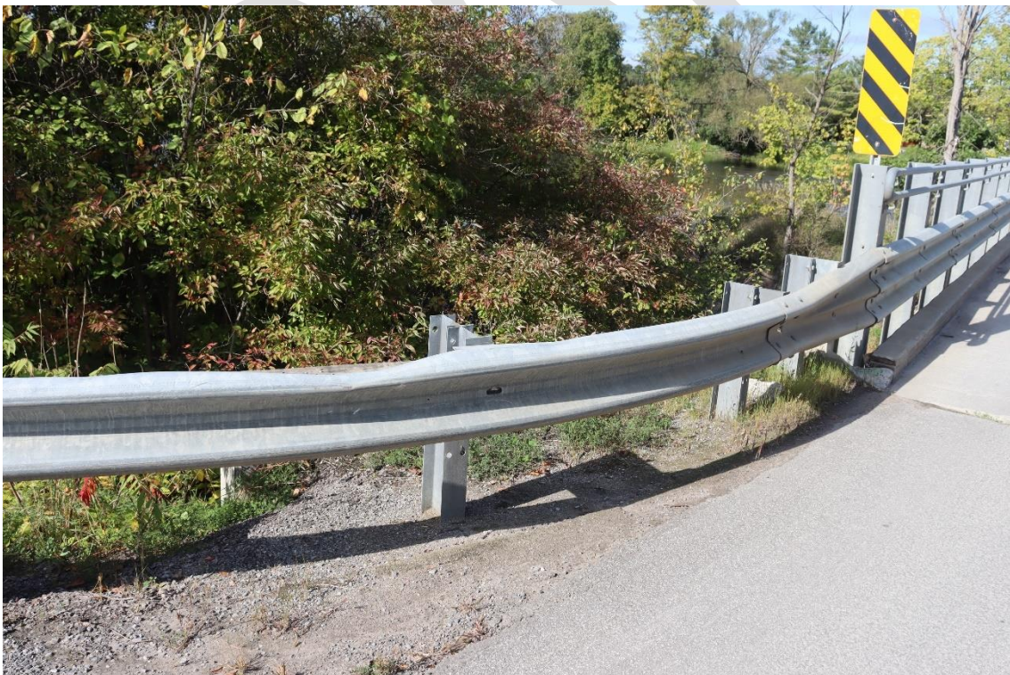
Image 4. South guide rail on east bridge
