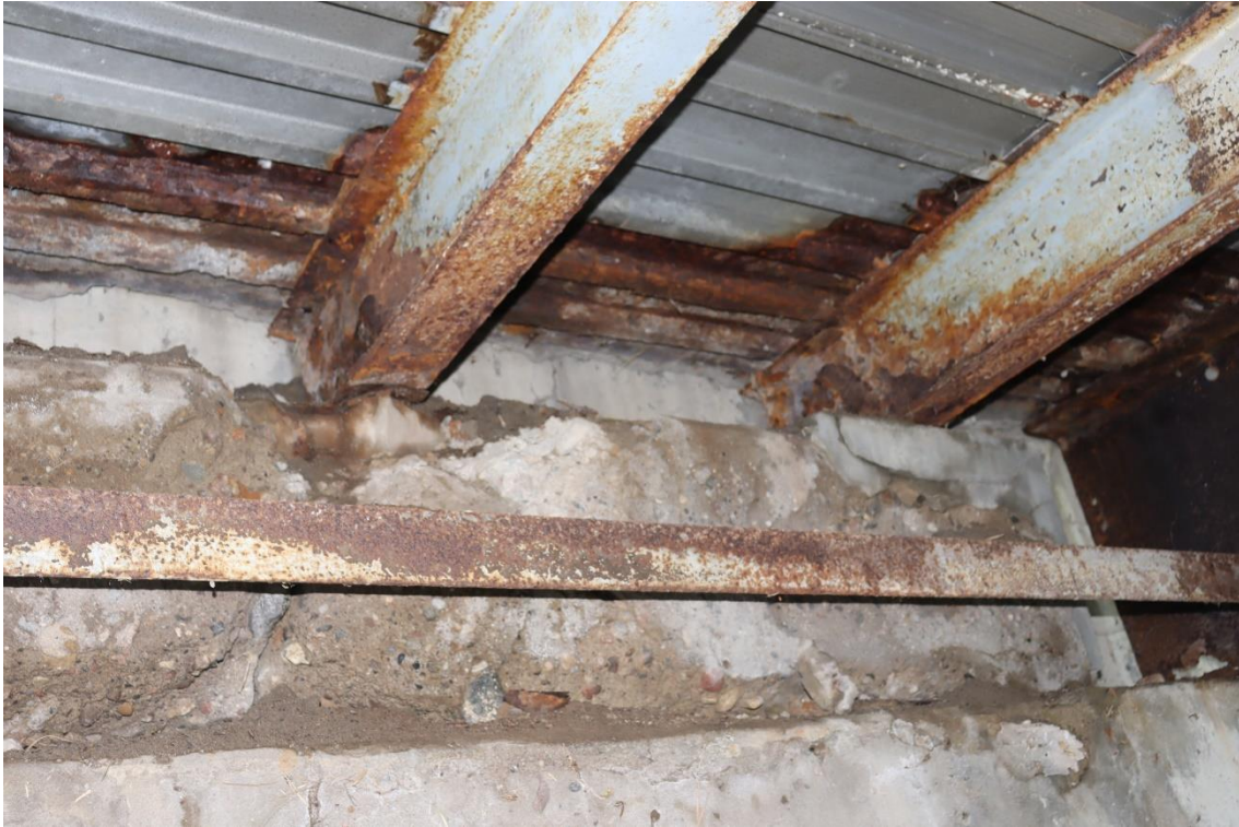
Image 53. General western bearing area of northern 2 stringers of west bridge
