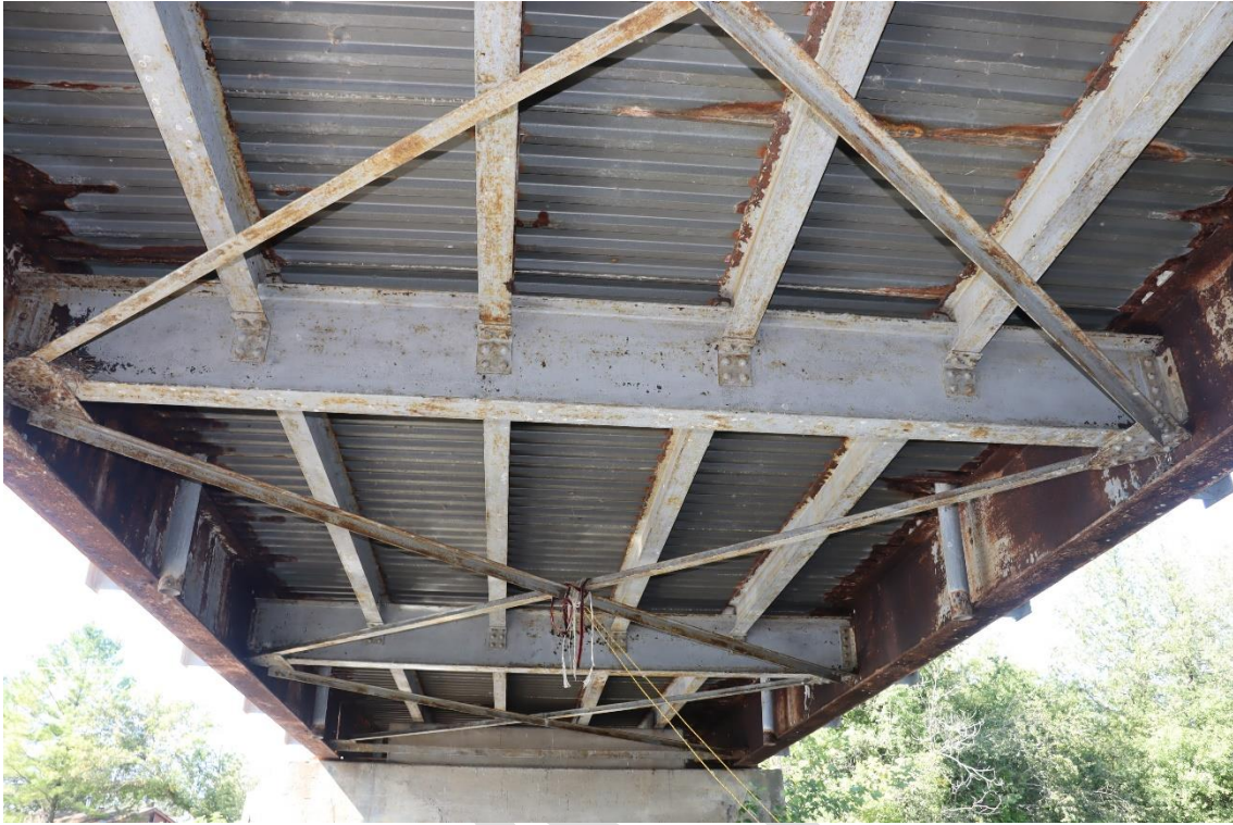
Image 21. Soffit & floor system of east span of west bridge facing west
