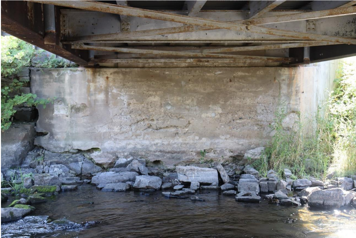
Image 7. East abutment of east bridge
