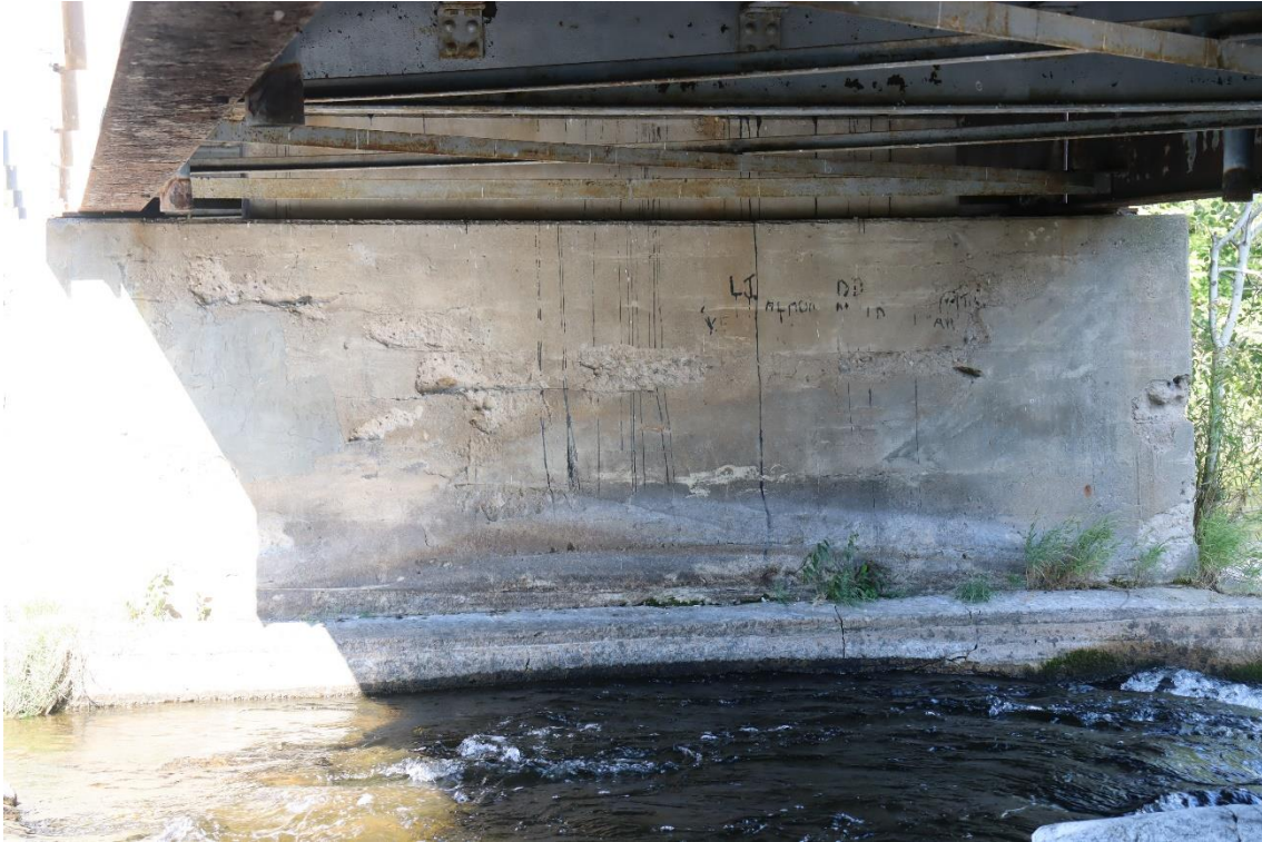
Image 10. East face of pier of middle bridge
