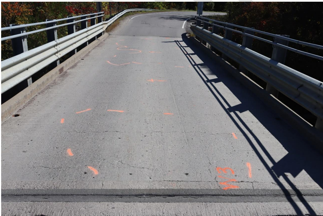
Image 31. East bridge deck condition survey
