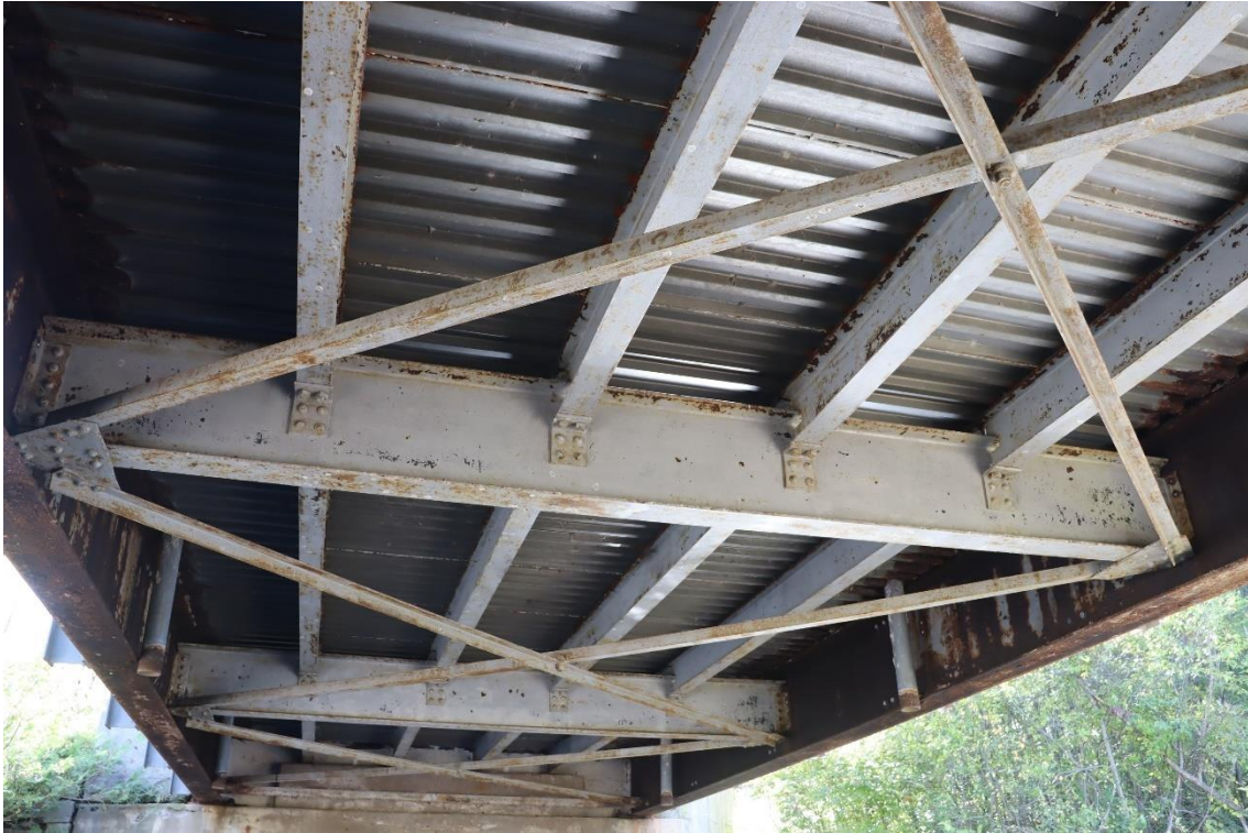
Image 9. Structural steel & soffit of east bridge facing east
