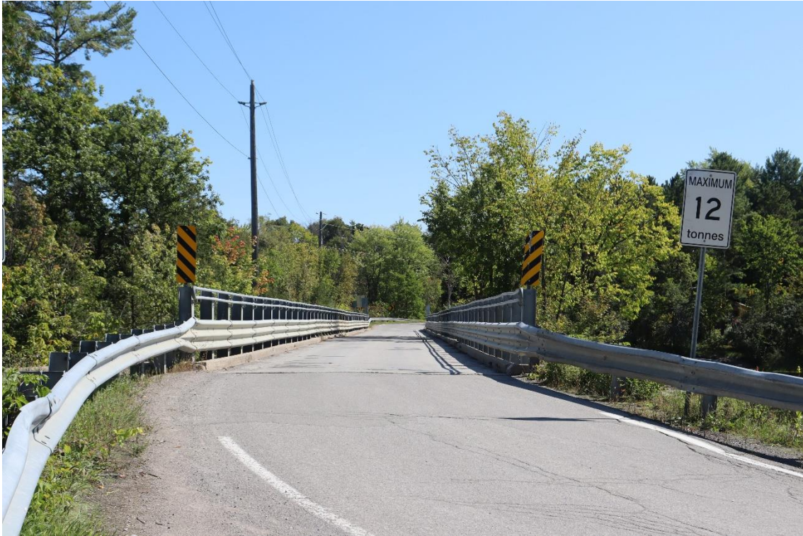
Image 19. West approach of west bridge
