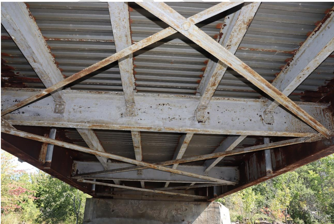
Image 16. Soffit & floor system of west span of middle bridge facing east
