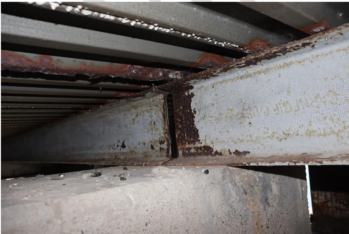
Image 48. Typ. stringer ends on pier of west bridge
