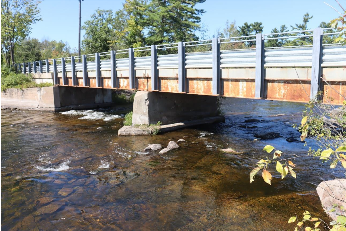
Image 17. South elevation of middle bridge
