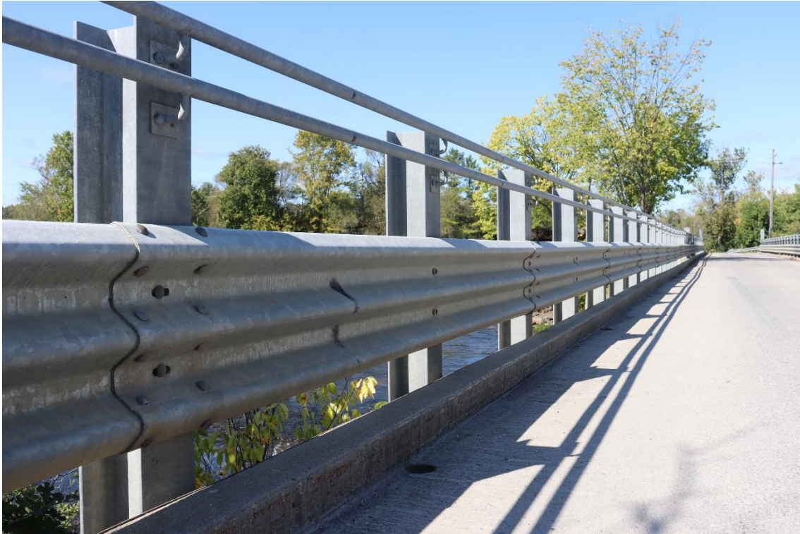
Image 19. Typ. guide rail on middle bridge
