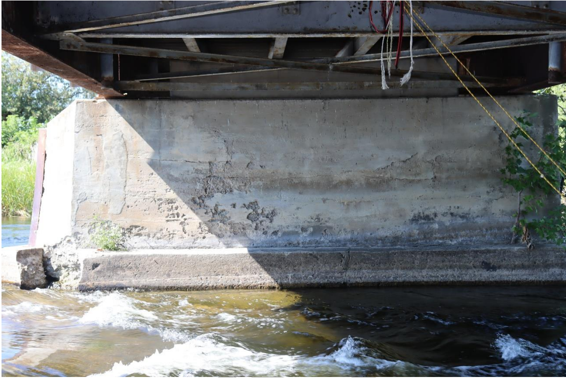
Image 24. East face of pier of west bridge
