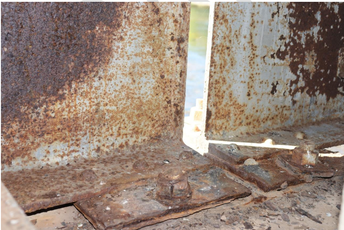
Image 11. Pier bearing of south girders of middle bridge
