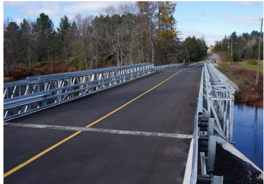
French Line Road Bridge- Lanark Highlands
