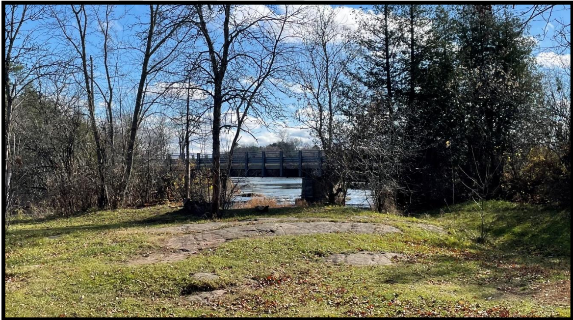
Figure 21: View towards the Blakeney Bridge from Blakeney Rapids Park. Source: Contentworks, November 2022.
