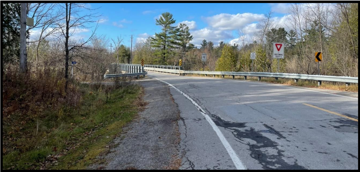
Figure 8: East approach to Blakeney Bridge, November 2022. Source: Contentworks.
