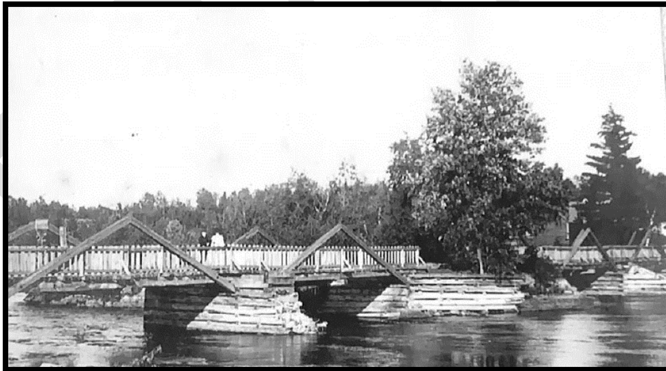
Figure 4: Timber bridge at Blakeney, [1900], looking towards the south (upstream) side of the bridge. Source: Ramsay Women's Institute, Tweedsmuir History Book 7 , accessed online at http://images.ourontario.ca/Partners/FWIO/FWIO003203526_0040p.pdf .
